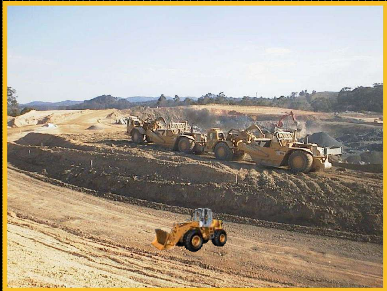
Roadwork, Pacific Highway
