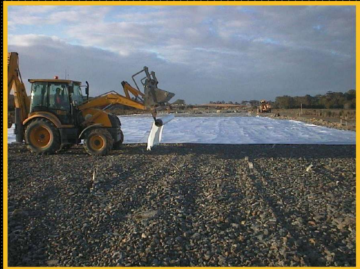
Geofabrics used on Pacific Highway
