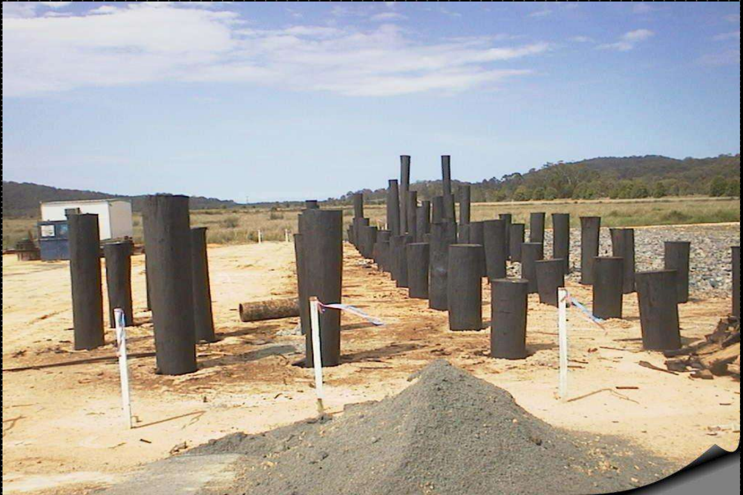
Driven timber piles, Pacific Highway
