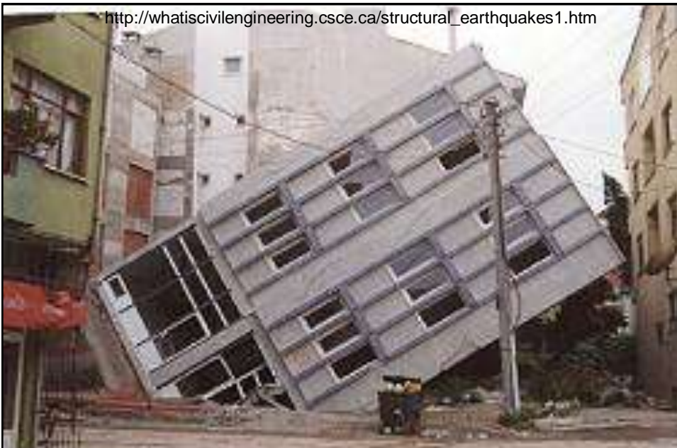
Overturning of a building due to liquefaction failure of the foundation soil during the Kocaeli earthquake, Turkey, August 17, 1999, Magnitude 7.4
