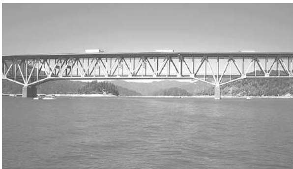
An example of a Warren truss (with verticals). See page 87.
