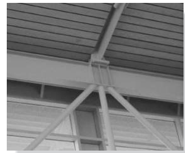
Diagonal bracing.
