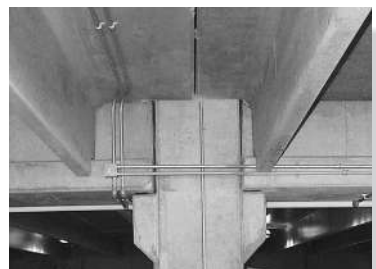
Concrete smooth or "roller" support.
