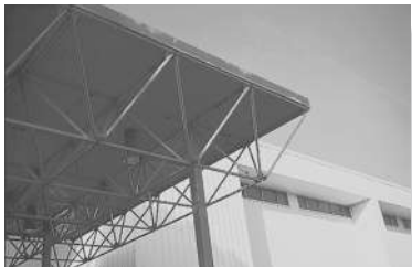
The roof of this pavilion is supported using a system of space trusses.
