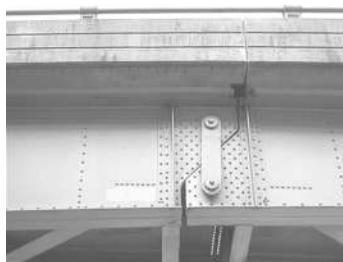
The short link is used to connect the two girders of the highway bridge and allow for thermal expansion of the deck.
