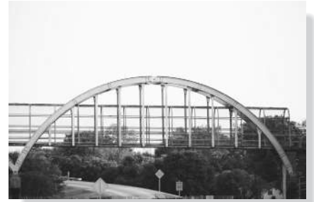
This three-hinge truss arch is used to support a pedestrian walkway. This bridge is referred to as a “through-arch bridge.”
