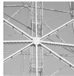
This gusset plate is used to connect eight members of the truss supporting structure for a water tank.
