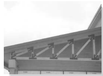
Gusset plates used for a wood truss.
