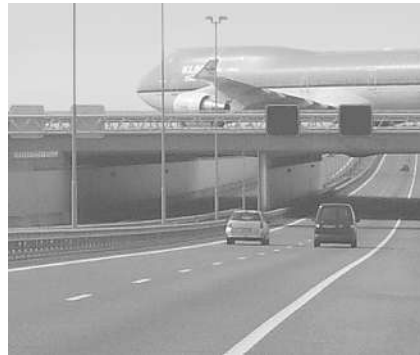
The girders of this bridge must resist the maximum moment caused by the weight of this jet plane as it passes over it.
