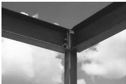
Pin-connected steel members.
