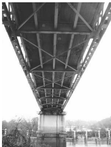
Stringers, floor beams, and cross bracing shown under a typical bridge.
