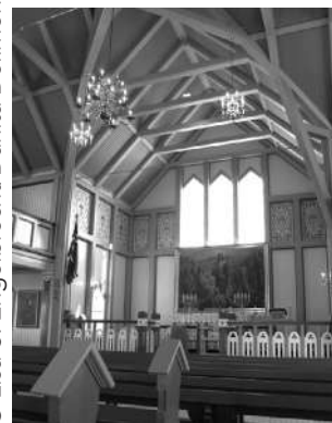
Timber frames having a variable moment of inertia are often used in the construction of churches.
