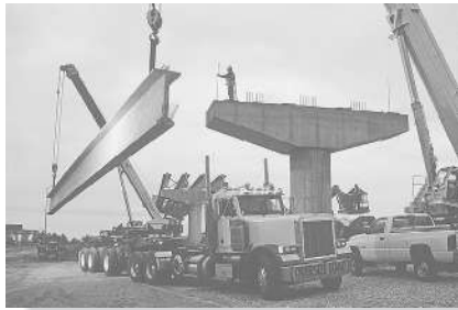
The tapered concrete hammerhead pier is used to support the girders of this highway bridge.
