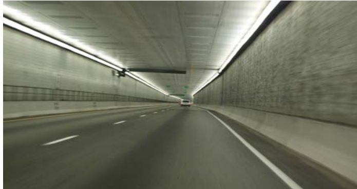
View from Inside the Eisenhower Tunnel
