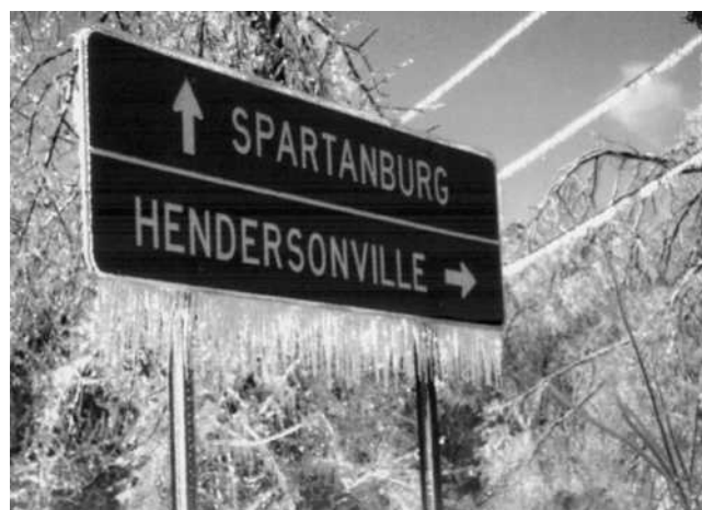
FIGURE C10.2-1 Glaze Ice Accretion Caused by Freezing Rain
