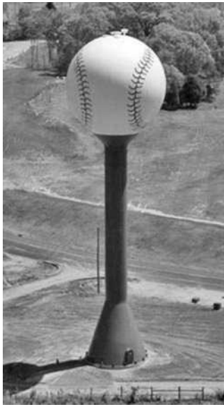
FIGURE C15.7-2 Small-diameter, single-pedestal steel tank
