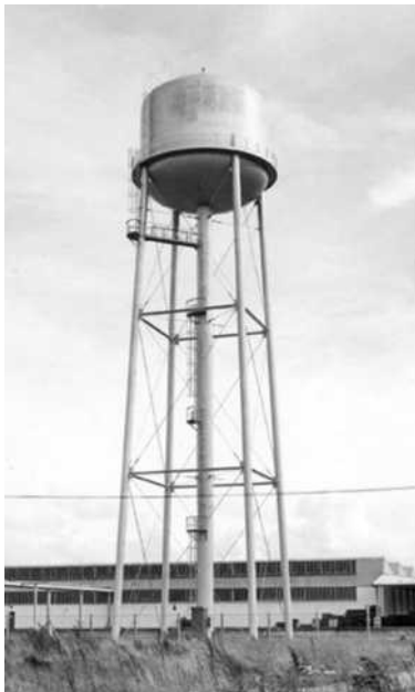
FIGURE C15.1-1 Steel multilegged water tower
