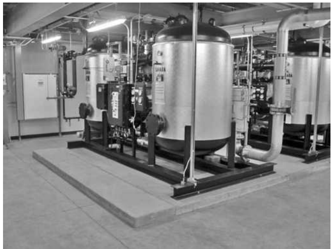
FIGURE C13.1-6 Skid-Mounted Components
