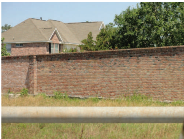
FIGURE C15.6-4 Typical Masonry Ground-Supported Cantilever Wall
