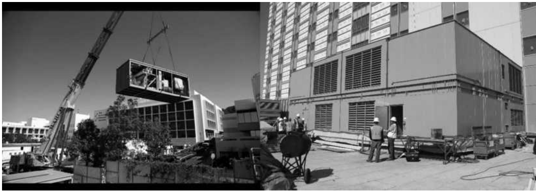
FIGURE C13.1-7 Premanufactured Modular Mechanical Systems
