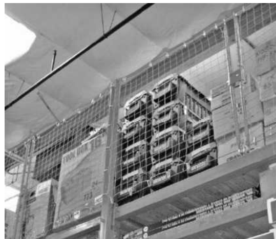
FIGURE C15.5-1 Merchandise restrained by netting
