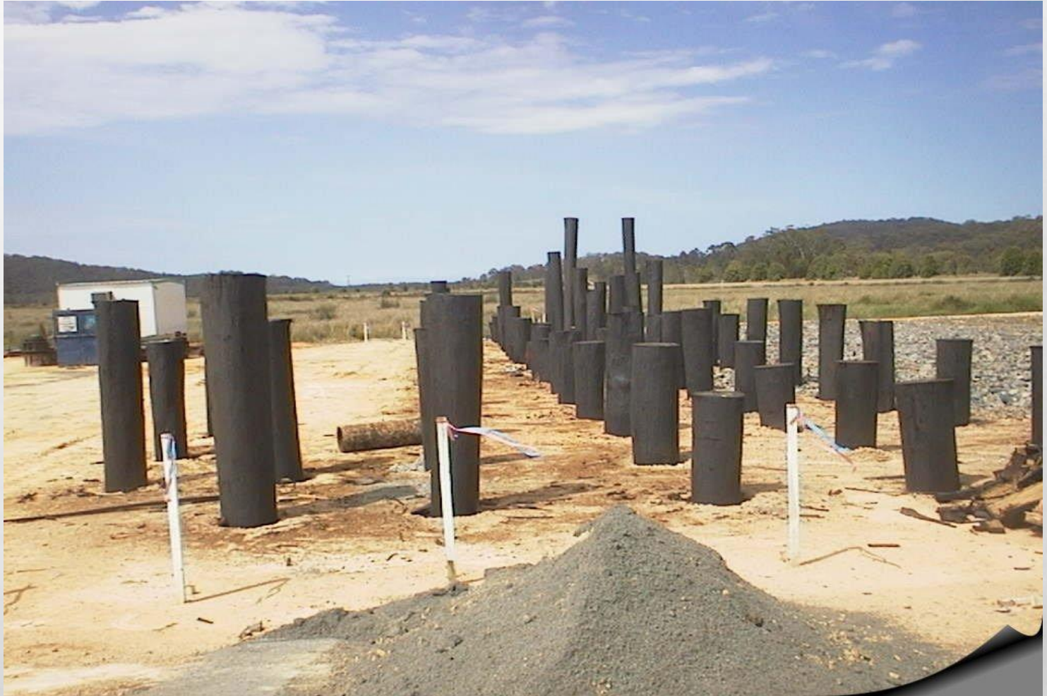
Driven timber piles, Pacific Highway
