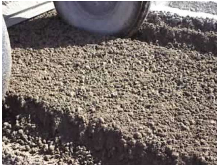
Lime flocculating clay
