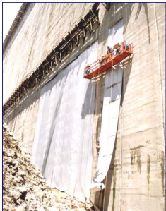
(Lining a Concrete Dam)
