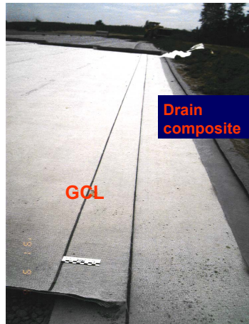
Capping of an old wastedump
