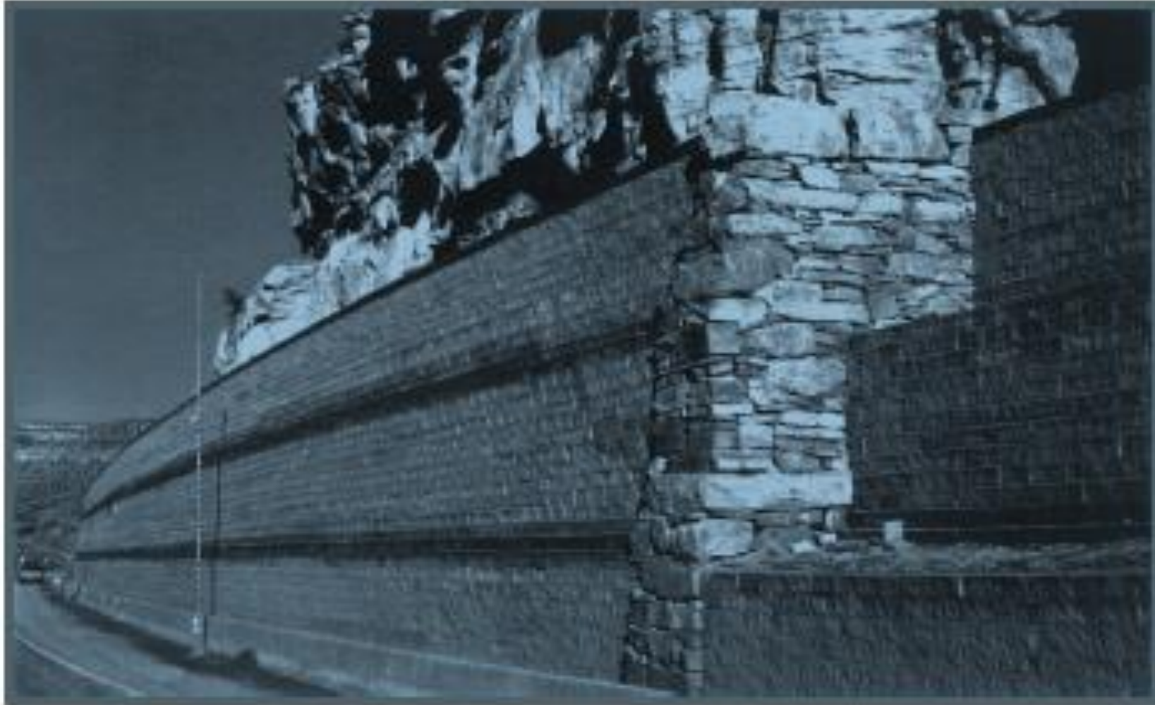
Figure 8.35 A completed geotextile-reinforced retaining wall in DeBeque Canyon, Colorado (Courtesy of Jonathan T. H. Wu, University of Colorado at Denver, Denver, Colorado)
