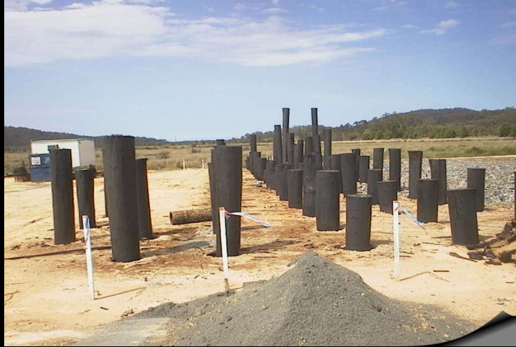
Driven timber piles, Pacific Highway
