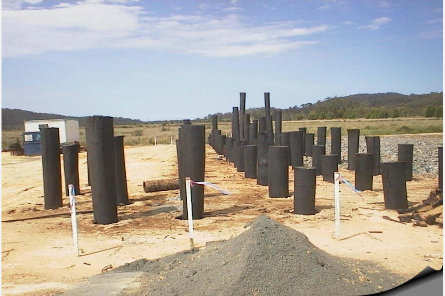
Driven timber piles, Pacific Highway
