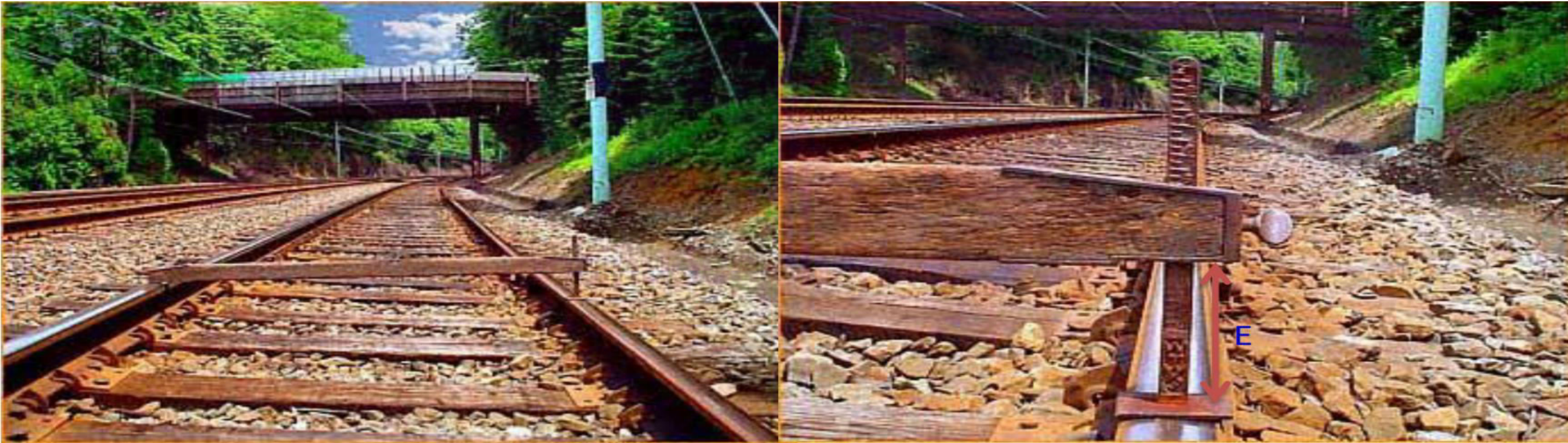
Track level in place indicating 5" of superelevation on the outside rail of a curve.
