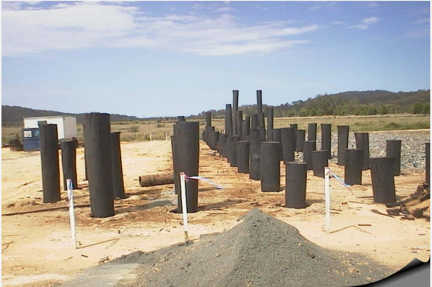
Driven timber piles, Pacific Highway
