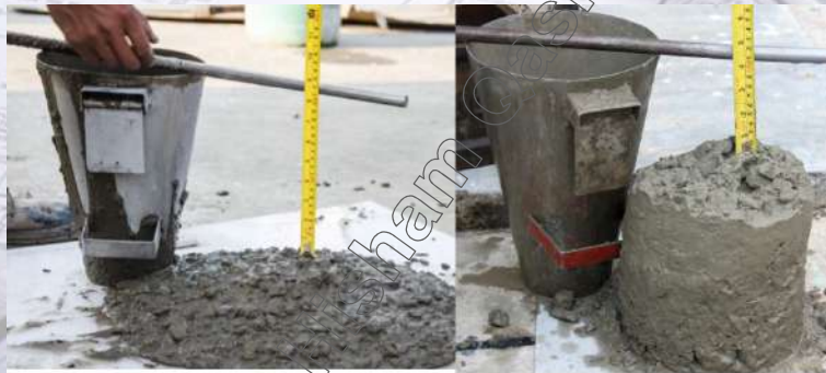
What Should Site Engineer Do If On-site Slump Test Fails?
