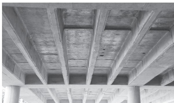
(b) Section X-X joist floor system
