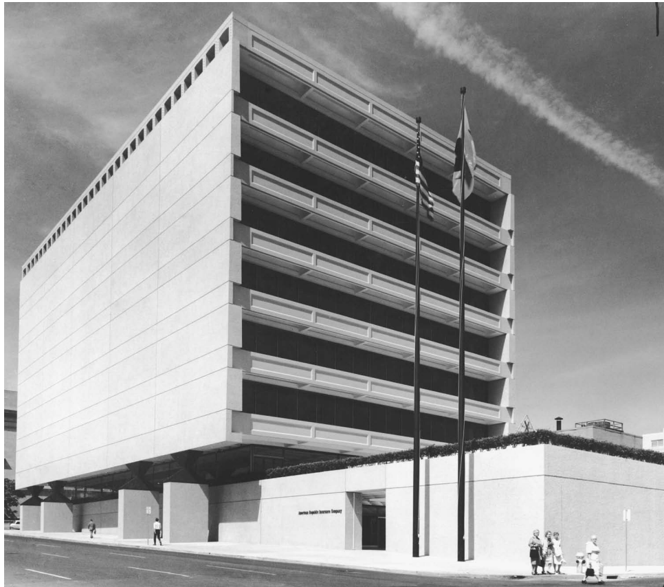
FIGURE 19.23 Precast girders with 99 ft span and 44 in. depth for a column-free interior. (Courtesy of Portland Cement Association.)
