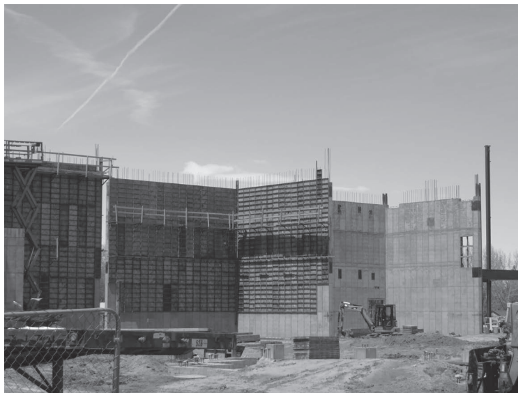
FIGURE 14.1 Bearing walls under construction. (Photograph by Charles W. Dolan.)
