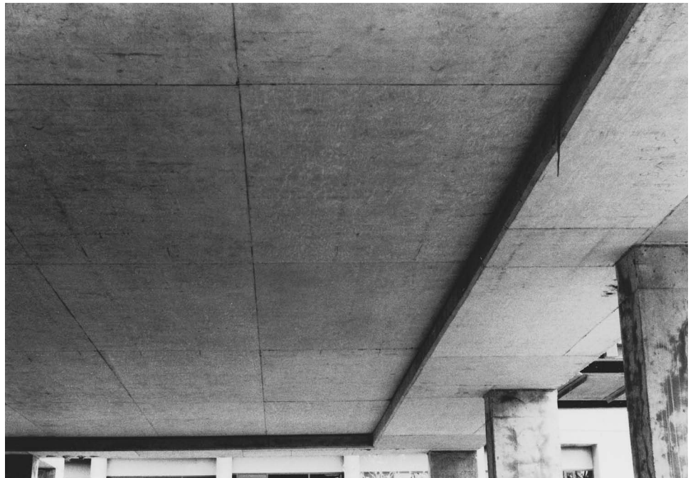
(b) Edge band at exterior column
