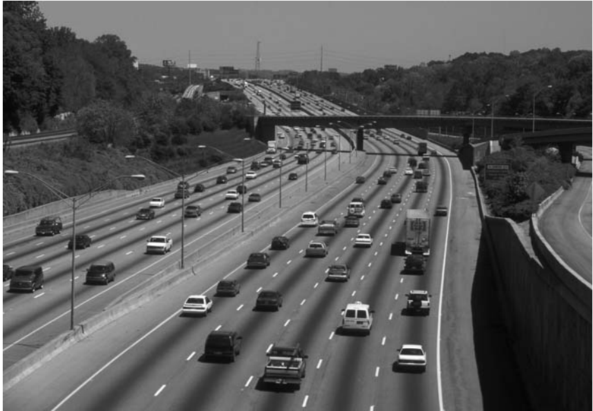
(a) Note how vehicles shy away from both roadside and median barriers, driving as close to the lane marking as possible. The existence of narrow lanes compounds the problem, making it difficult for two vehicles to travel alongside each other.
