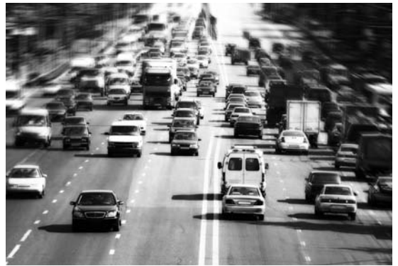
(d) Undivided multilane highway in a suburban environment.
