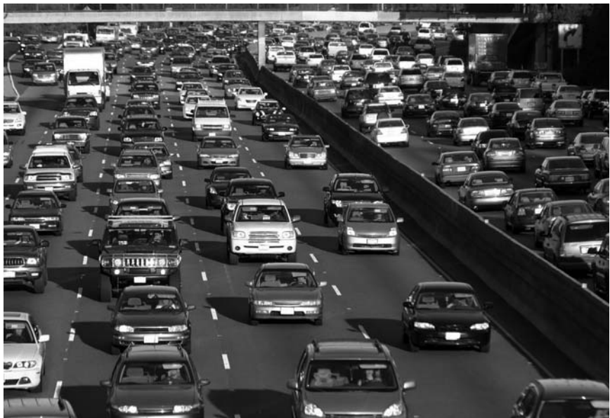
(b) In this case, vehicles shy away from the roadside barrier. This causes the placement of vehicles in each lane to be skewed toward the median. This is also an indication that the median barrier illustrated here does not present an obstruction to drivers.
