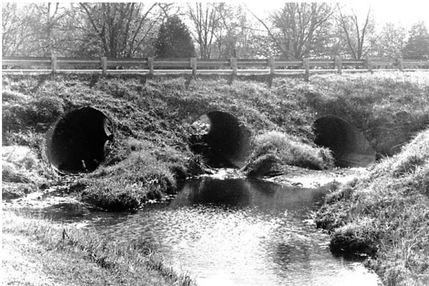
(a) Corrugated metal arch culvert (ARMCO)
