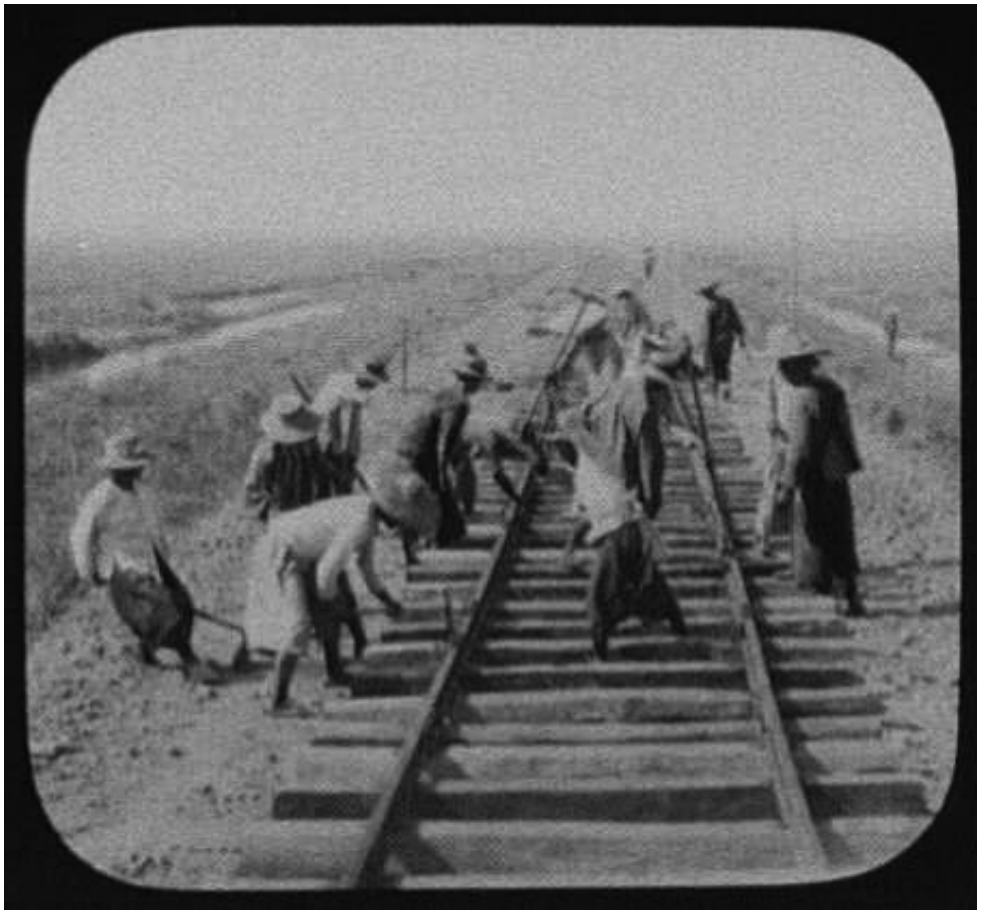
Figure 1.2 Workmen Repairing Railroad Track—1895
