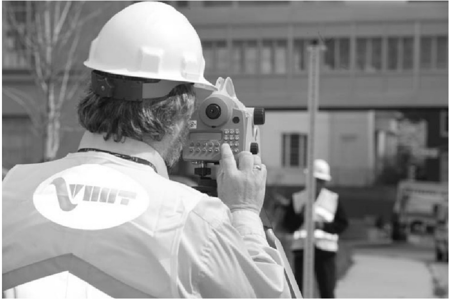
Figure 14.4(d) High-Accuracy Digital Leveling Using a Trimble DiNi 12 Digital Level
