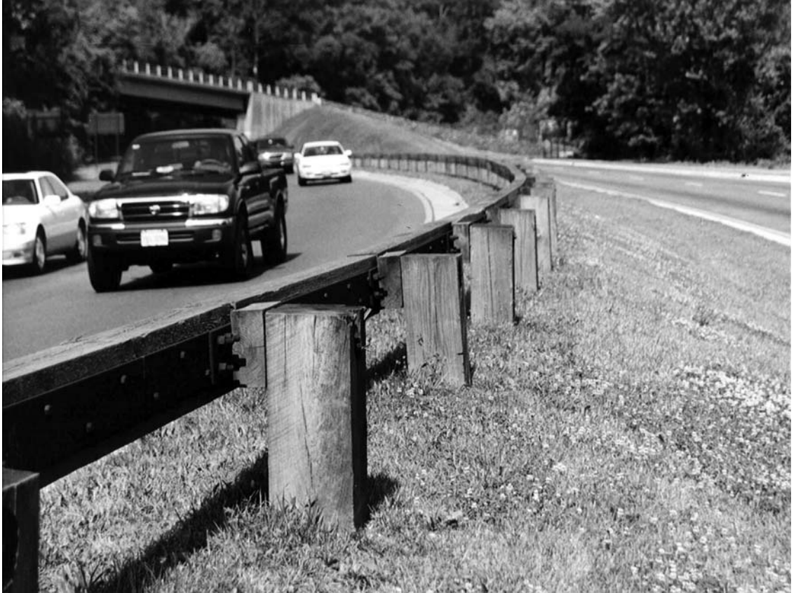
Figure 15.6 Steel-Backed Timber Guardrail
