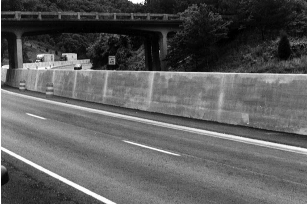
Figure 15.7 Single-Slope Concrete Median Barrier
